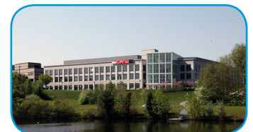
JCVI 15,000 square feet 9605 Medical Center Drive New office and lab space by converting lab space
