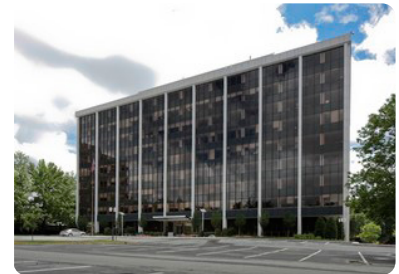
George Washington University renewed at 6116 Executive Boulevard for 29,263 square feet.
