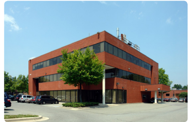
SABR Biologics, 1600 East Gude Drive - 10,000 sf to build GMP compliant contract manufacturing space.
