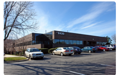
CellPhire, 9430 Key West Avenue - 5,500 sf of office and lab space for needed growth.
